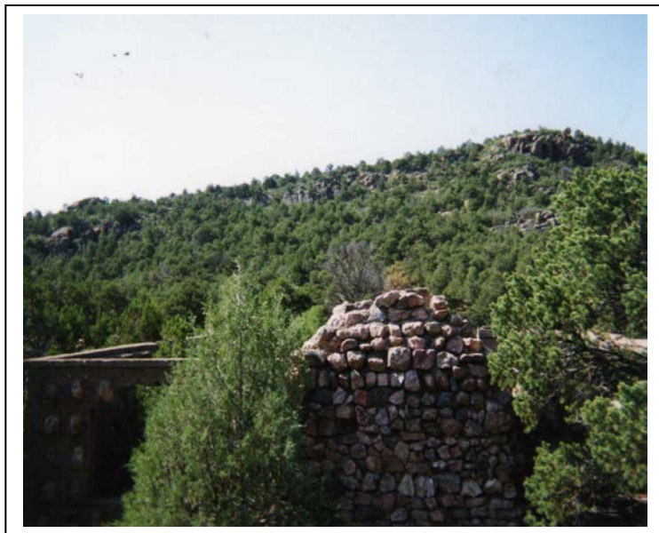
The back of the Vista Lodge fireplace previous to the fire in 2013.
