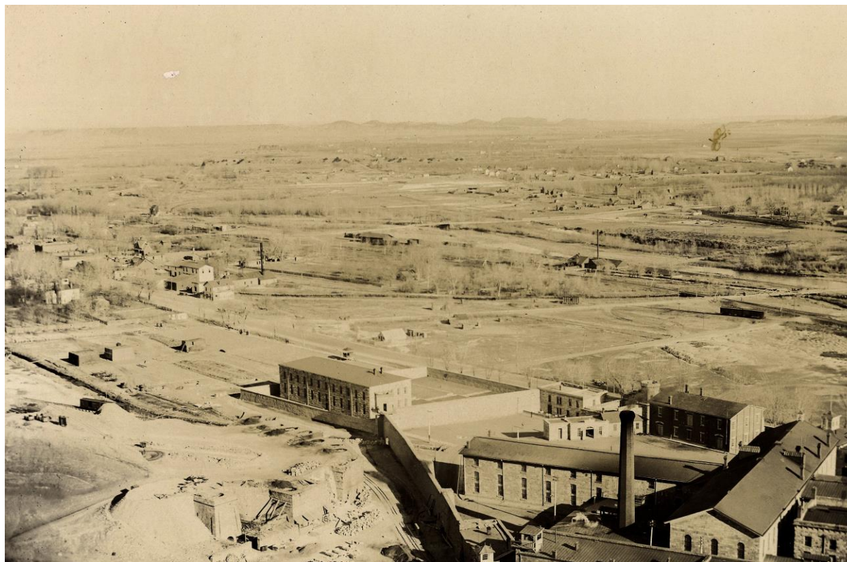
The view from the "Hog Back" in 1886 towards the East side of Canon City, including the penitentiary.
