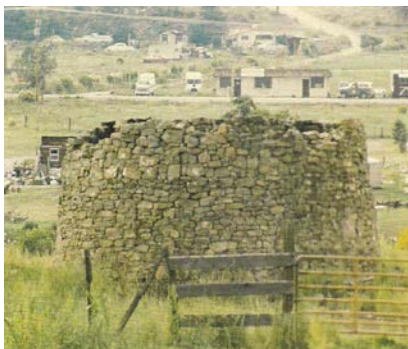
PRIOR TO DEMOLISHING BY BULLDOZER, ONE OF THE HOWARD KILNS
