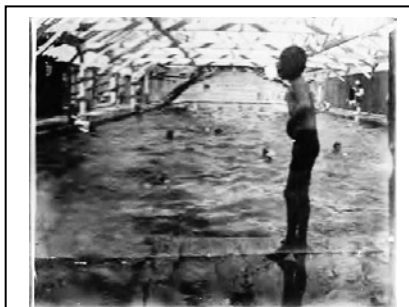
ROOF OVER THE POOL
